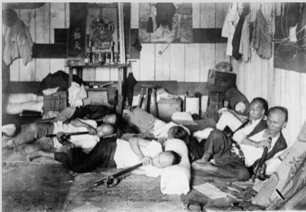
Figure 2. Opium den on Malinta Street, Manila.
